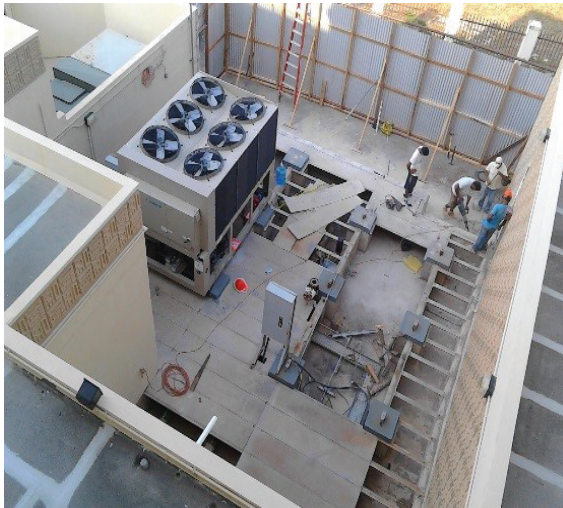
The installation of the HVAC System 2016
